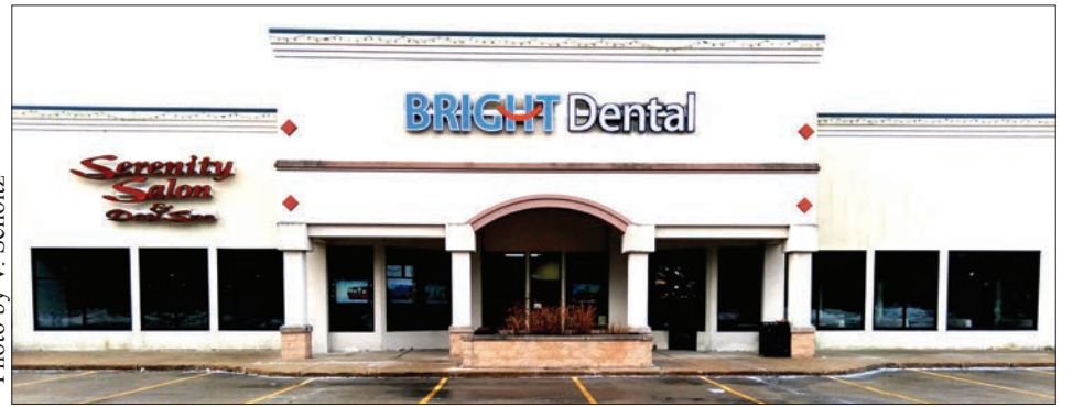
Bright Dental exterior facing Northport Drive
