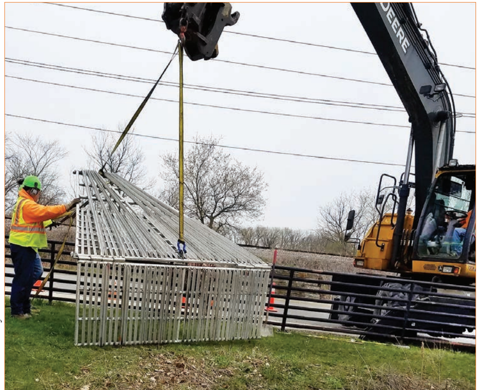
City workers installing the carp gate at Warner Pond.
